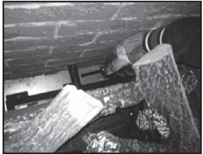
Figure 1. Air Shutter Location
