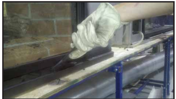
Figure 14.5 Inserting Glass Clip Tool
