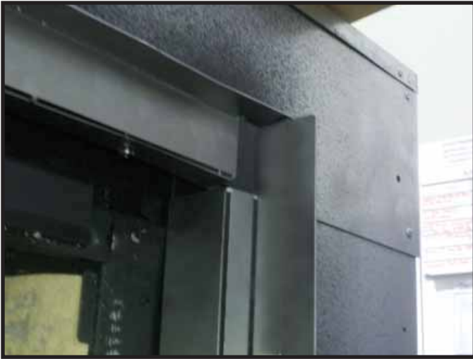
Figure 13.4 Finishing Template Bends - Inoperable (Fixed) Doors
