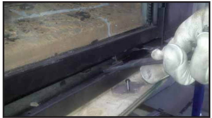
Figure 14.4. Glass Clip Tool Location
