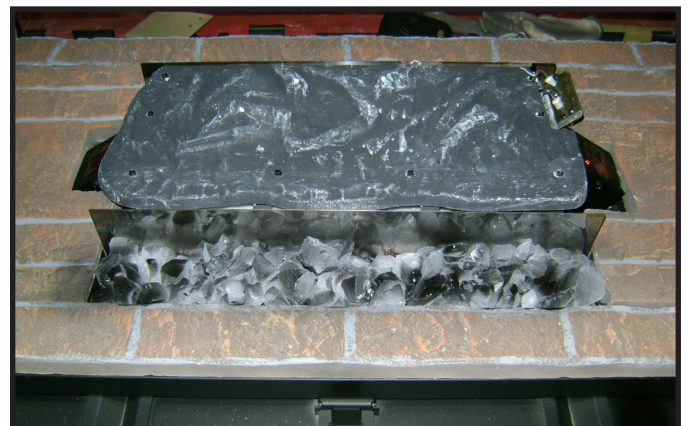
Figure 11.16 Finished Ember Bed
