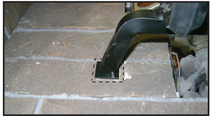
Figure 3. Grate leg placement.
