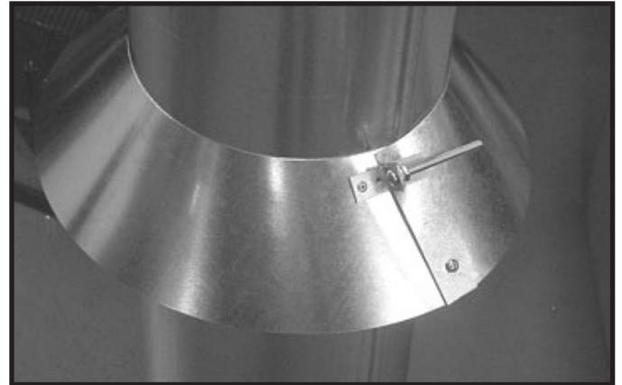
Figure 7.12 Insert Bolt into Brackets
