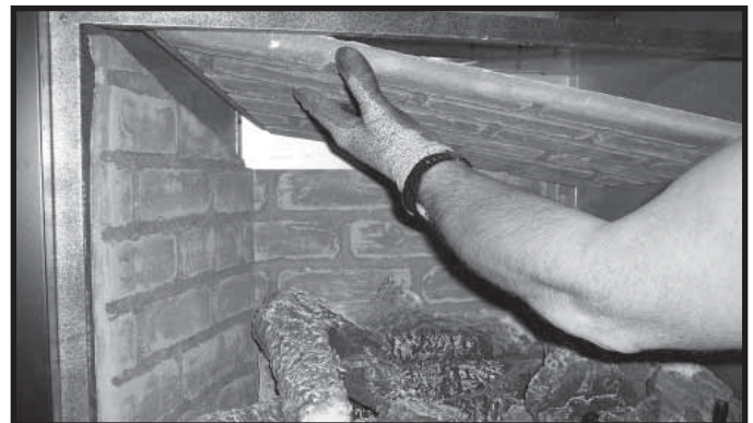
Figure 7.10 Remove Top Refractory
