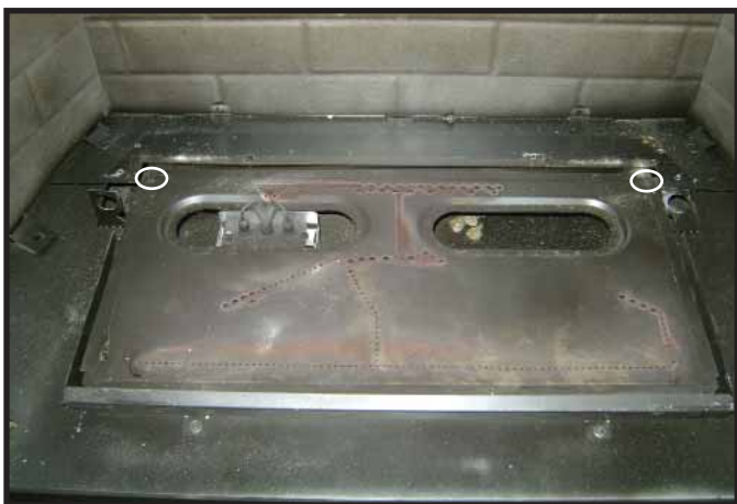
Figure 3.8 Remove Screws from Burner Assembly Rear Corners
