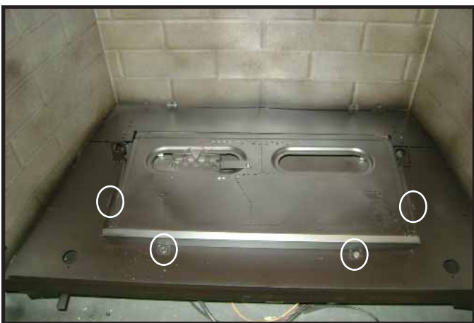
Figure 3.9 Remove Burner Skirt
