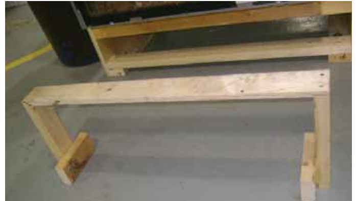
Figure 1.4. Field-Constructed Appliance Support
