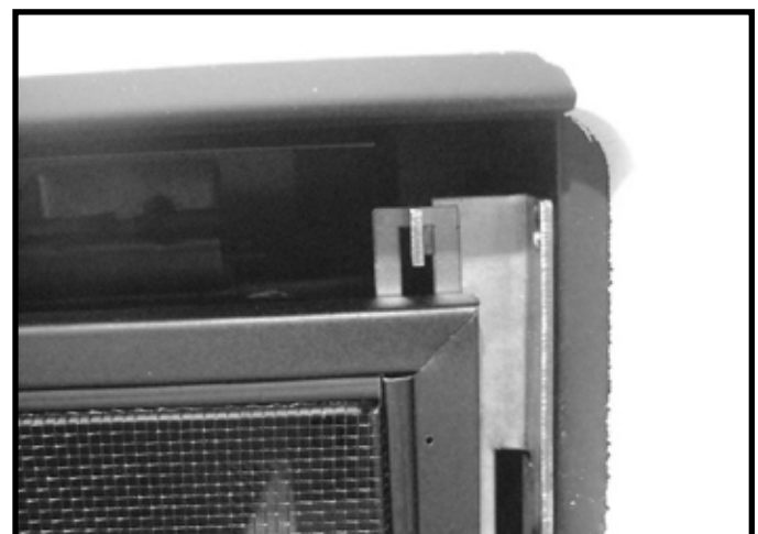
Figure 3. Mesh Installed.
