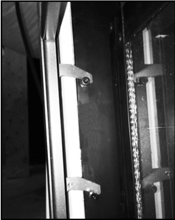
Figure 4. Bracket Engagement with Bolts
