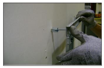
Figure 4.6 Installing Anchors in Hollow Wall
