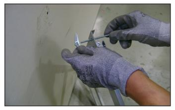
Figure 4.5 Toggle Bolt Installation through Mounting Bracket
