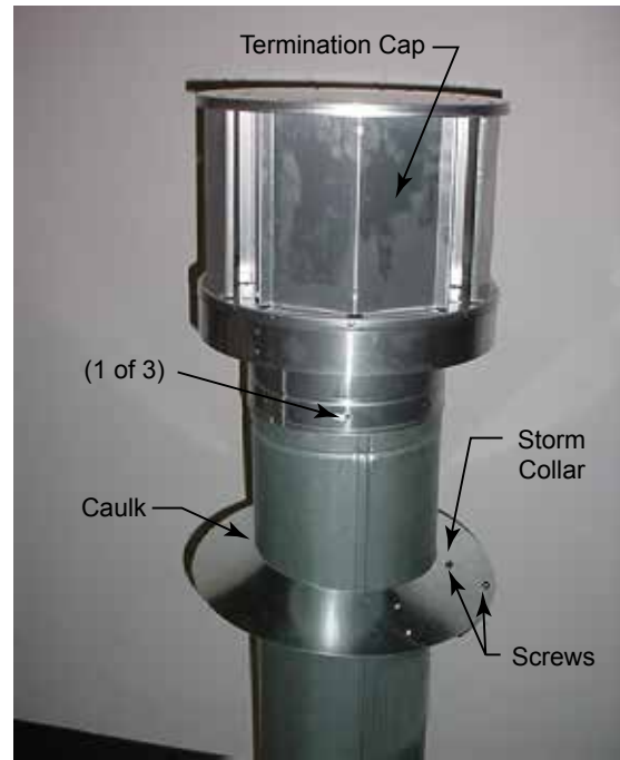
Figure 63 – Secure with Screws
