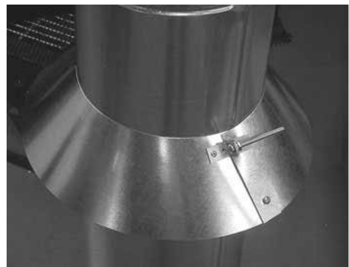
Figure 62 – Insert Bolt into Brackets
