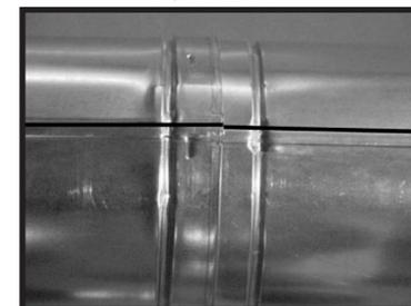
Figure 7.4 Joints INCORRECT
