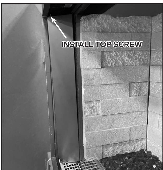
Figure 11.21 Transition Panel installed
