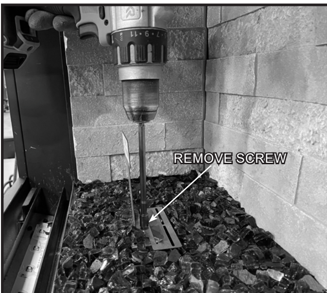
Figure 11.4 Place Media, Remove Media Placement Jig Screw
