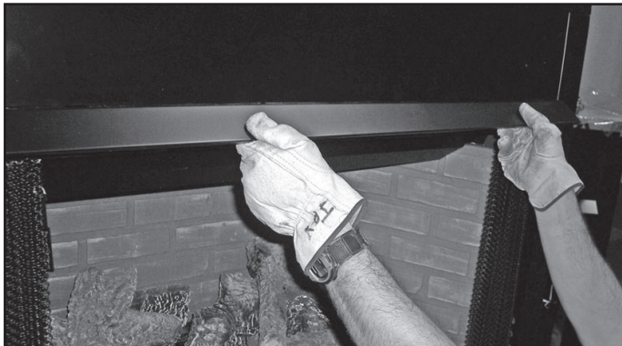
Figure 14.27 Installation de la hotte
