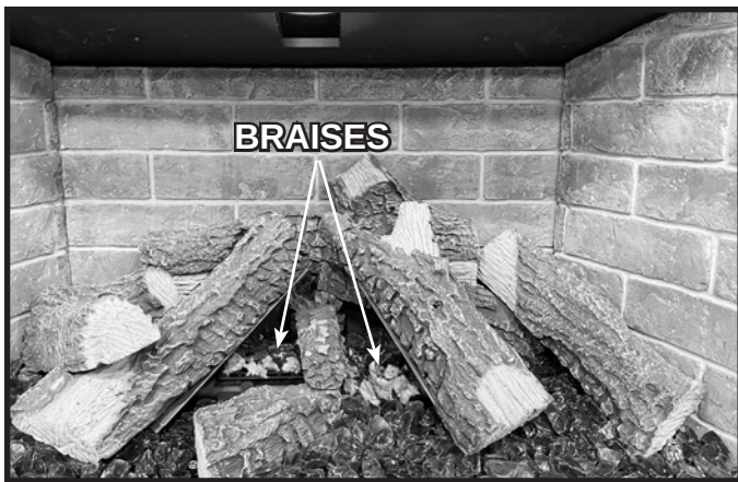
Figure 21 Bûches de chêne, support et Glowing Embers (braises incandescentes) installés
