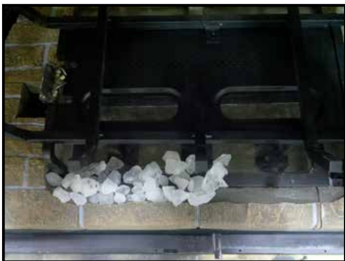
Figure 14.1. Installation de Teco-Sil
