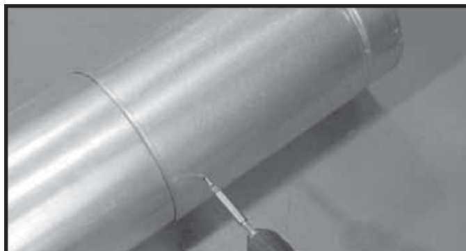
Figure 10.7 Vis de la section coulissante
