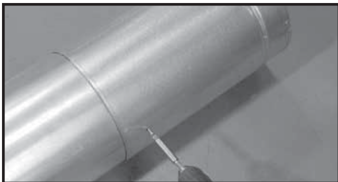
Figure 10.7 Vis de la section coulissante
