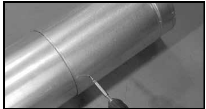
Figure 10.6 Vis de la section coulissante
