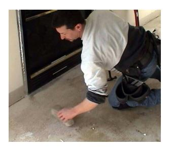
3. Make sure that the floor area in front of the fireplace is level and clean, and has minimal flex.
