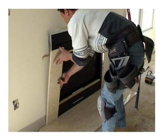
5. Now set the stone legs in position on the hearth, on either side of the fireplace, adjusting for fit. Apply the silicone adhesive in 3 or 4 places on the back of the legs and push them against the wall, making sure that the **polished** edges face toward each other and the fireplace. For faster silicone set up, pull the leg back / away from the wall and allow the silicone to "string". Wait 30 seconds and re-position leg.
