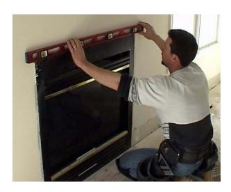
Ensure the fireplace is installed plumb and level. The face flushes with the outer surface of the wall. Correct any problems before proceeding. (It is a good practice to inspect the top of the firebox for trash or other combustible materials and remove them.)
