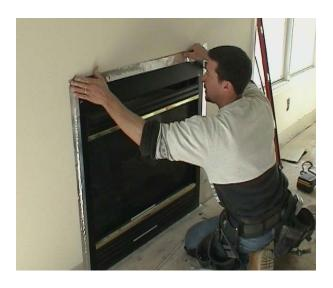
2. (Optional step.) In regions with extreme temperature variations adding an additional thermal barrier is recommended. With aluminum duct tape, tape around the firebox sealing the opening between the drywall and the firebox. (Available at local hardware stores.)
