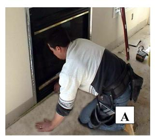
4. A. Measure and mark off the area around the firebox to determine where the hearth is going to fit on center. This will provide the area in which to lay the thin set. Following the "thin set" or mortar instructions, spread the mortar so that it extends to all the corners. Using a 3/8" trowel, trowel out the mortar allowing it to fully support the hearth. B. Lay hearth. C. Shimming should not be necessary using thin set.
