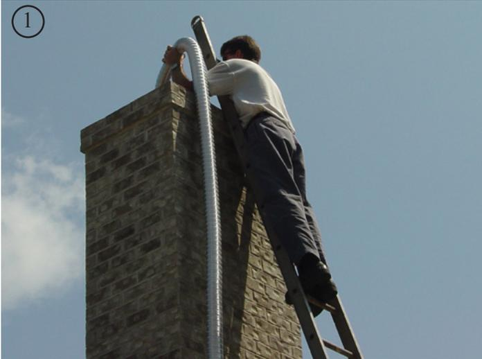
1 Feed chimney liners down the chimney and through the damper. If the fireplace opening does not allow enough room to connect the flue liners to the stove it is necessary to separate the exhaust/ intake pipe adapter from the stove body.
