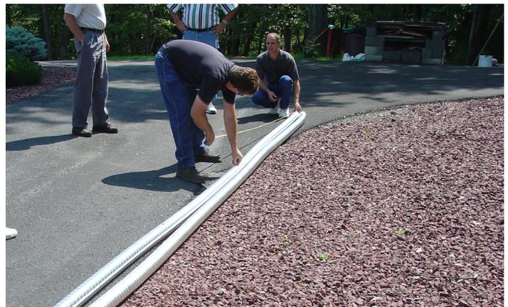
Uncoil the three inch aluminum chimney liners on the ground and measure to make sure the pipes are long enough. Mark one of the liners at both ends with paint and use it for the exhaust side connection. Once they are in the chimney it allows easier identification of intake and exhaust connections.
