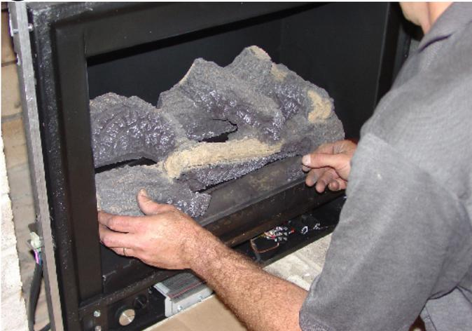
Place log set in firebox. Center the logs right to left and push back against the log stop.
