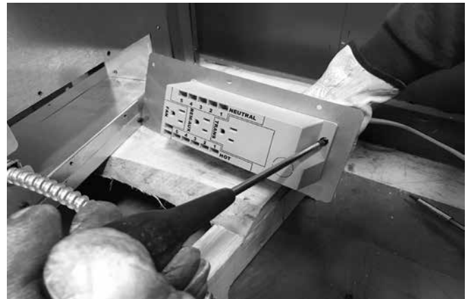
Figure 8.6 Junction Box Removal
