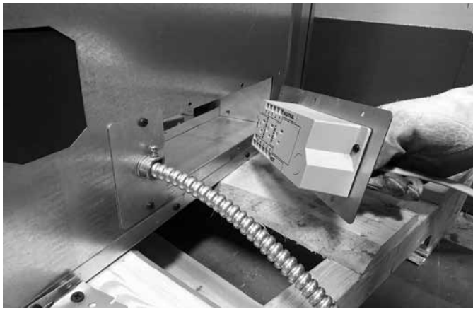
Figure 8.5 Junction Box Assembly
