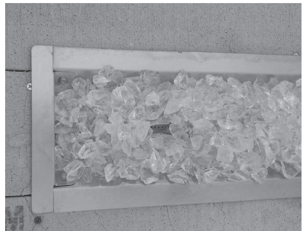
Figure 5.3 Pan Installed on Top of Finish Material
