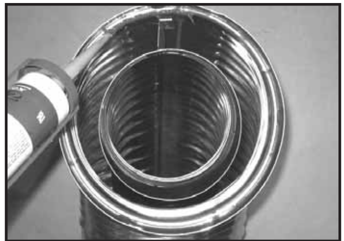
Figure 10.2 High Temperature Silicone Sealant (149 °C minimum continuous exposure rating)
