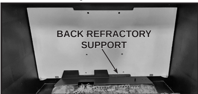
Figure 5 Back Insulation Board Installed
