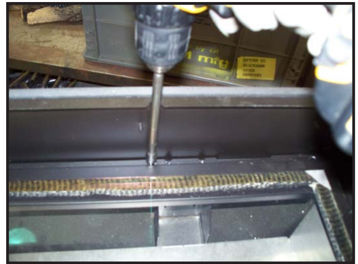
Figure 9.4. Gas and Electrical Access - Remove Glass Window
