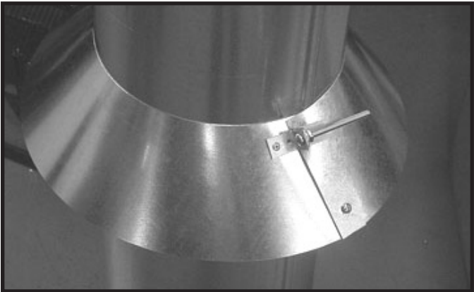
Figure 7.11 insert Bolt into Brackets
