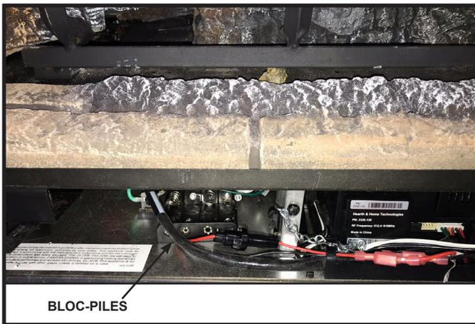
Figure 6.3 Bloc-piles installé
