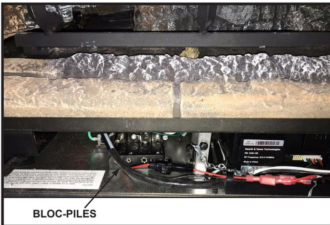
Figure 3.8 Bloc-piles installé
