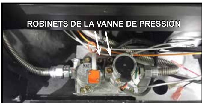
Figure 9.1. Robinets de la vanne de pression.
