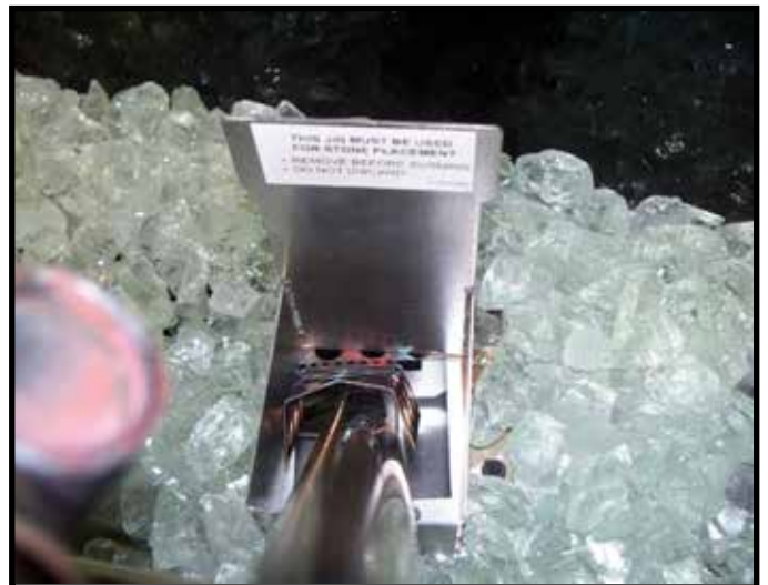
Figure 11.15 Retirer le support de placement des pierres
