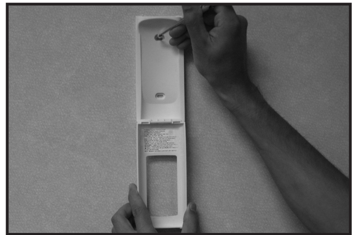
Figure 10.4 Mounting Remote Control Housing
