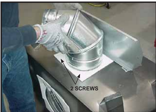
Figure 23. To attach the first section of flue pipe, make sure to use the fiberglass gasket to seal between the first vent component and the outer heater wrap. Use 2 self tapping screws to secure the gasket to the outer wrap.
