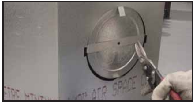
Figure 25. Cut the metal retaining band and fold the sides out.
