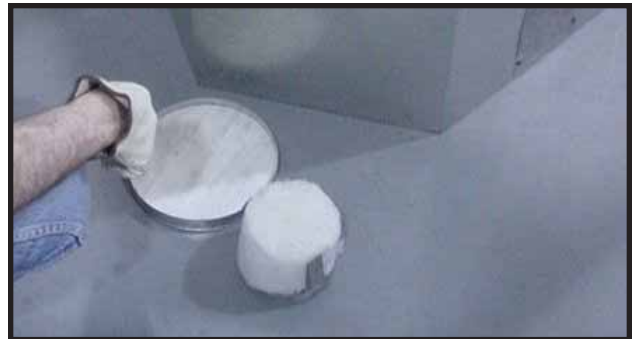
Figure 27. Discard the flue cap, remove and discard the insulation basket. Note: Once the flue cap has been removed it CANNOT be reattached.
