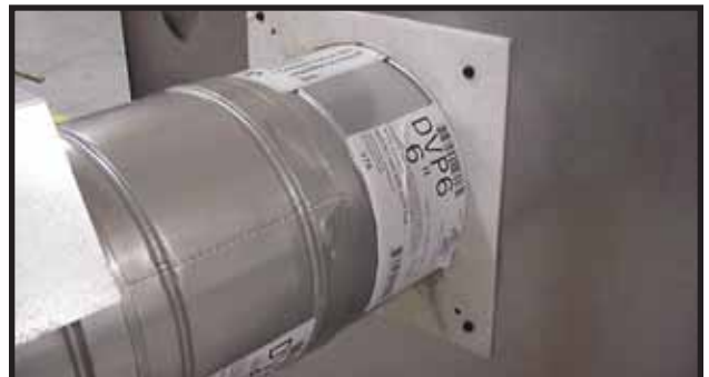
Figure 28. Attach the first flue section (it will snap into place). Slide the insulation gasket onto the flue section, up against the appliance and over the tabs. Use two self-tapping screws to secure gasket to outer wrap.
