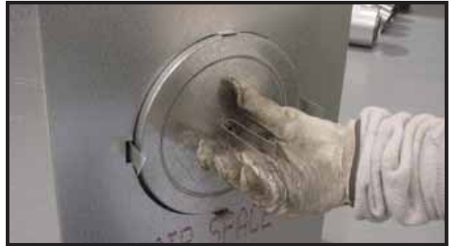
Figure 26. Fold the center parts of the retaining band out and use to remove the flue cap.
