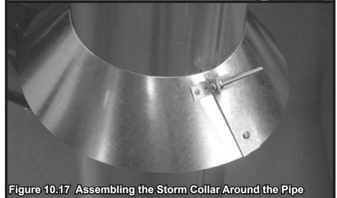
Figure 10.16 Assembling the Storm Collar
