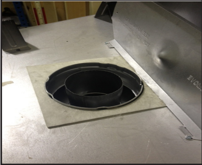
Figure 9.1 Rotate the top heat shield to the vertical position as shown above. The heat shield must remain in the vertical position.
