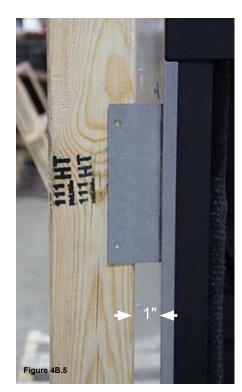
The nailing tabs will ensure the 1" minimum clearance is kept to combustible framing. Refer to Figure 4B.5
