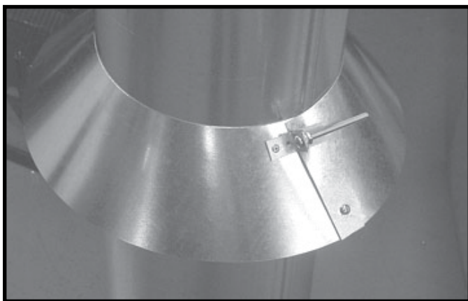
Figure 7.13 insert Bolt into Brackets
