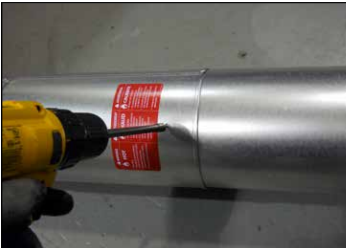
Figure 7.4 - Screws into Slip Section
