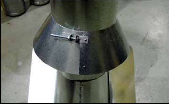
Figure 7.14 - Insert Bolt into Brackets
