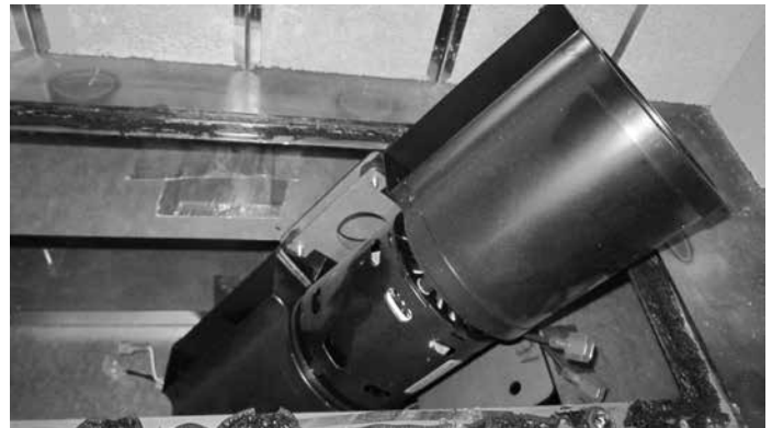
Figure 4.14 Remove Fan from Access Hole
