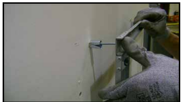
Figure 5 Installing Anchors in Hollow Wall
