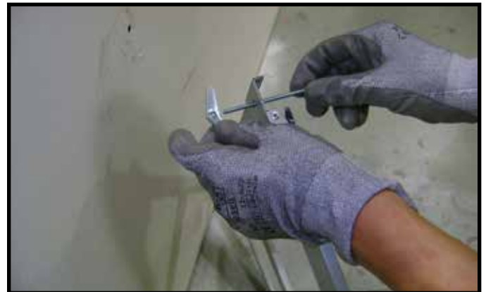
Figure 4 Toggle Bolt Installation through Mounting Bracket
