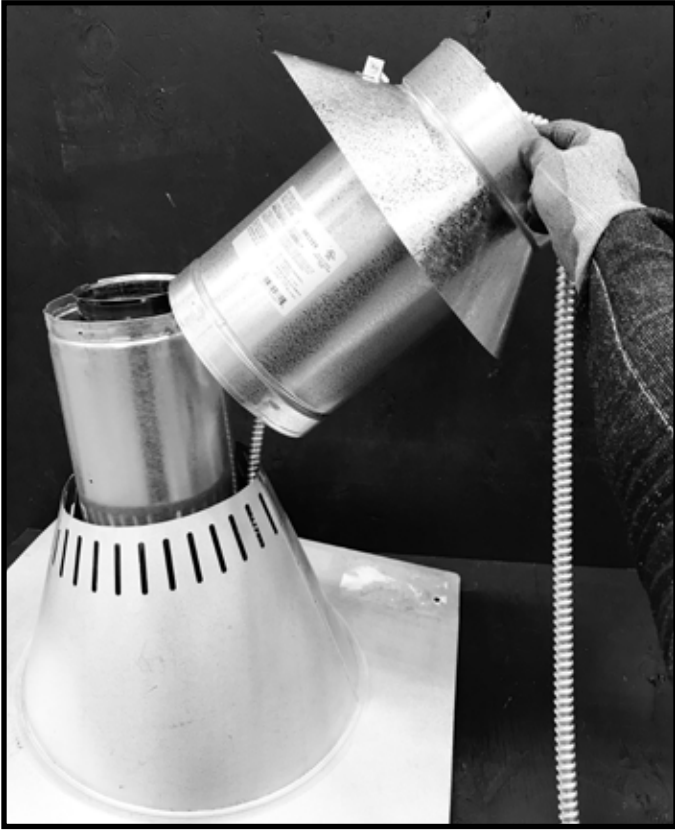
Figure 3.19 Route PVI Harness Through Flashing
