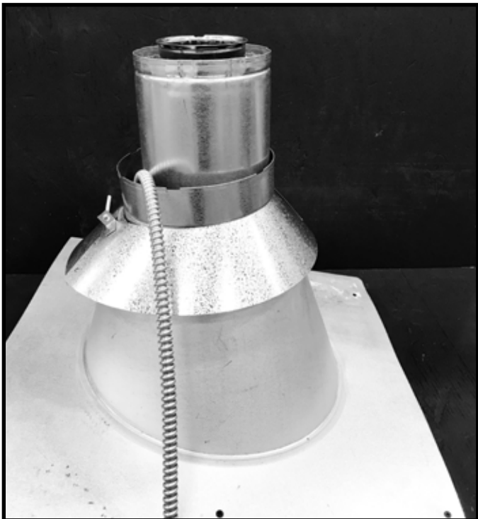
Figure 3.20 Storm Collar Resting on Flashing
