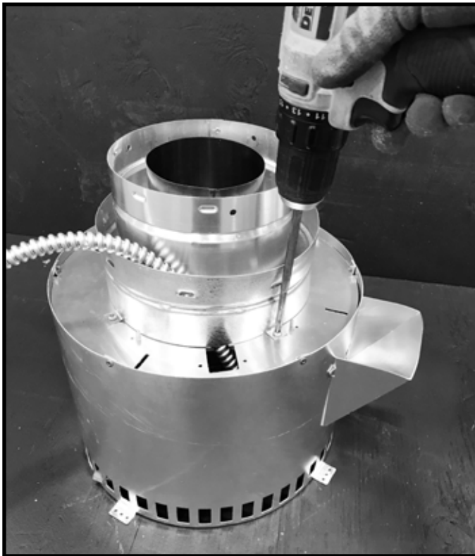
Figure 3.11 Attach Starting Collar
