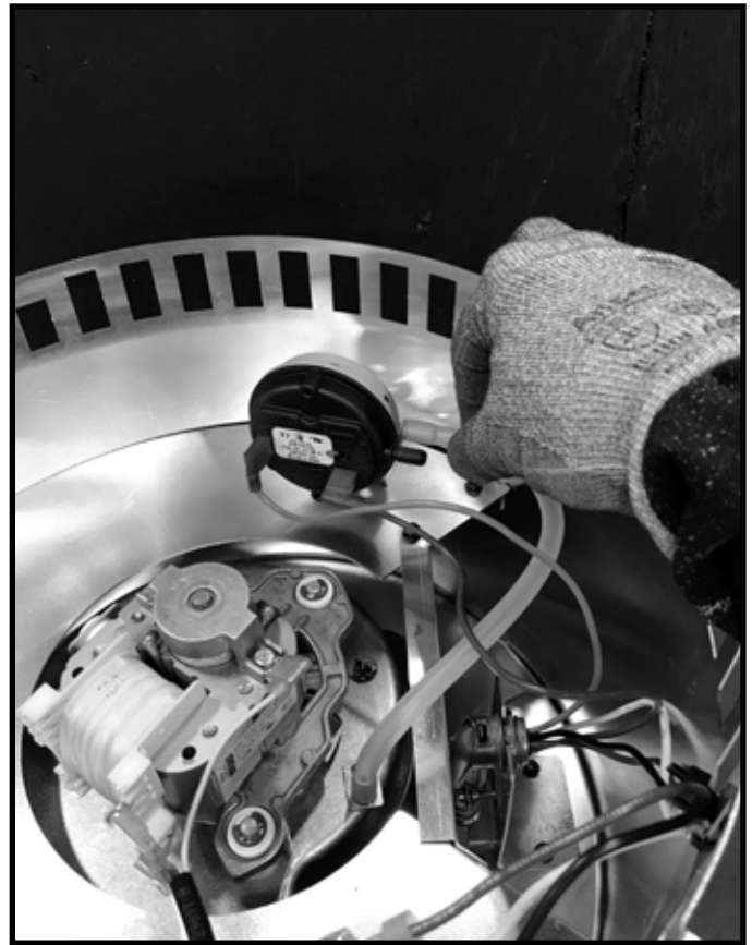
Figure 5.2 Remove Teflon Tubing
