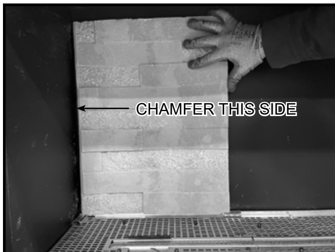
Figure 30 Position Back Left Refractory Panel - Architectural Stone
