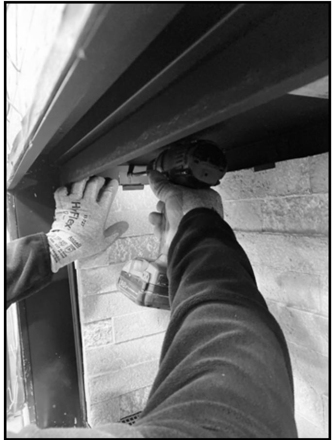
Figure 28 Install Side Refractory Panel Bracket with Screw
