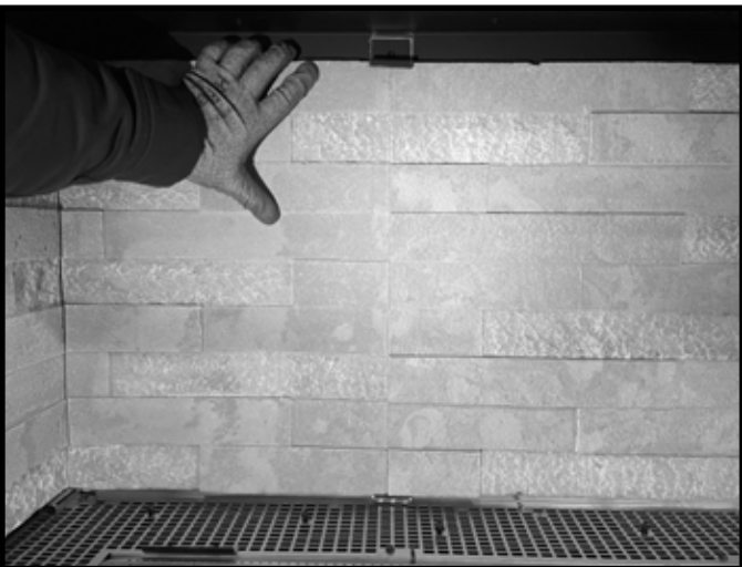
Figure 35 Refractory in Place and Positioned to Minimize Gaps
