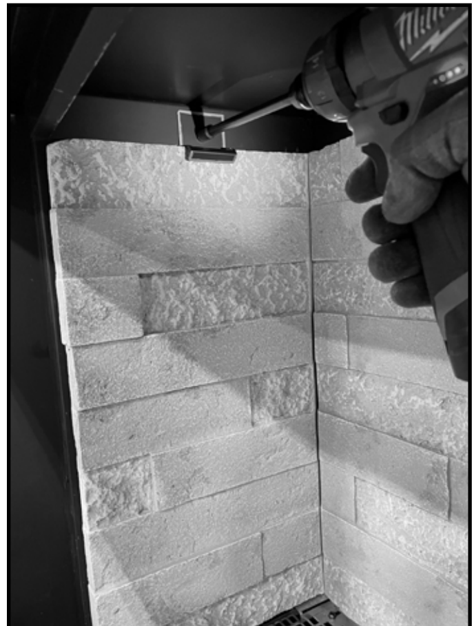
Figure 32 Install Left Side Refractory Panel
