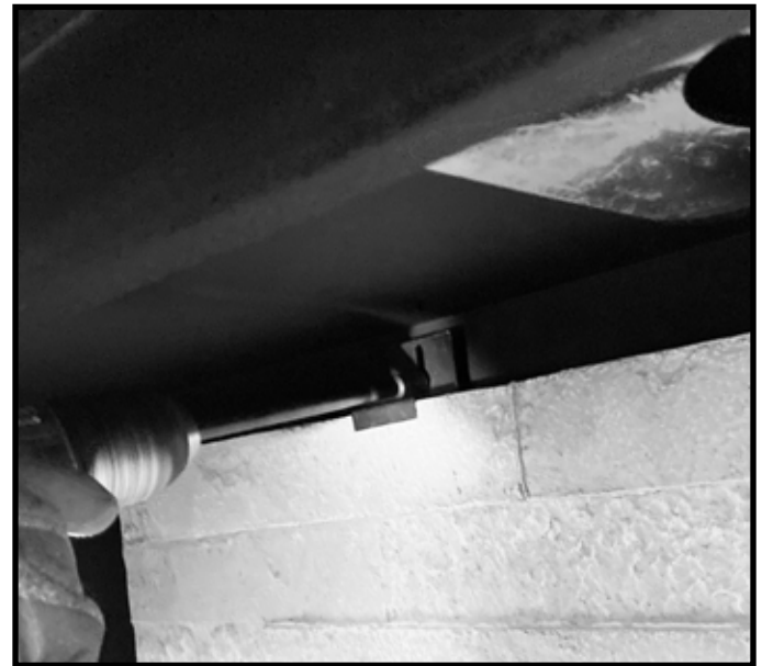
Figure 22 Install Refractory Brackets
