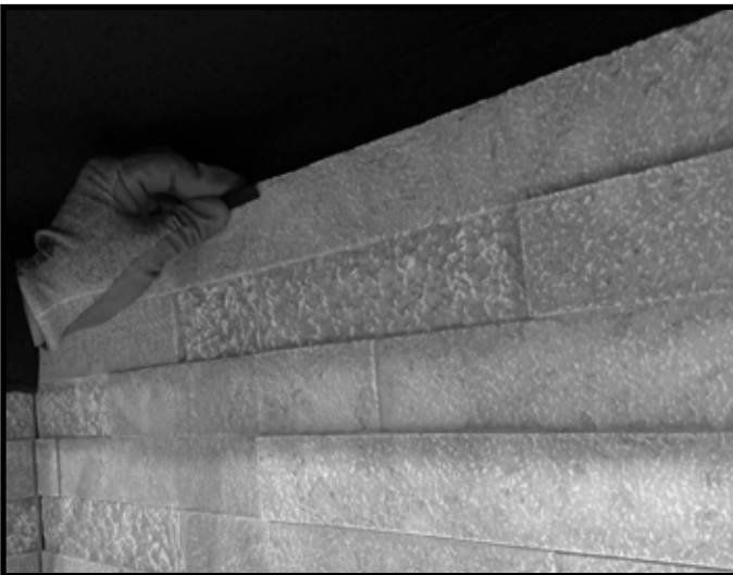
Figure 34 Install Refractory Brackets on Back Panel Seams
