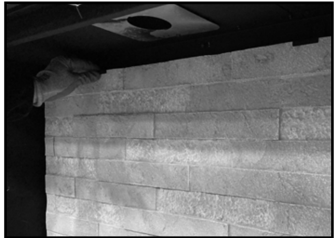
Figure 21 Position Refractory Brackets on Back Panel
