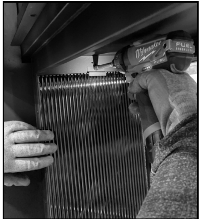
Figure 18 Install Side Panel Refractory Bracket
