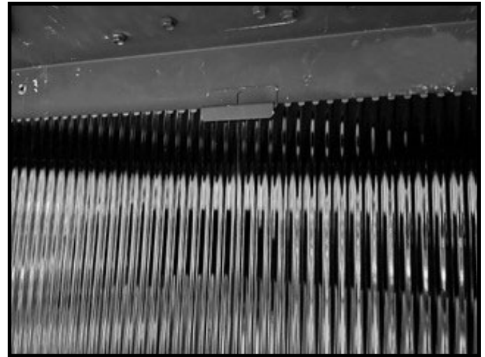
Figure 20 Install Refractory Brackets on Back Panel Seams
