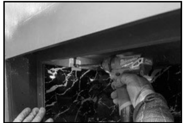
Figure 14 Install Refractory Bracket
