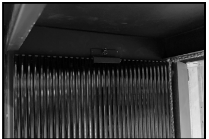
Figure 10 Side Refractory and Bracket Installed
