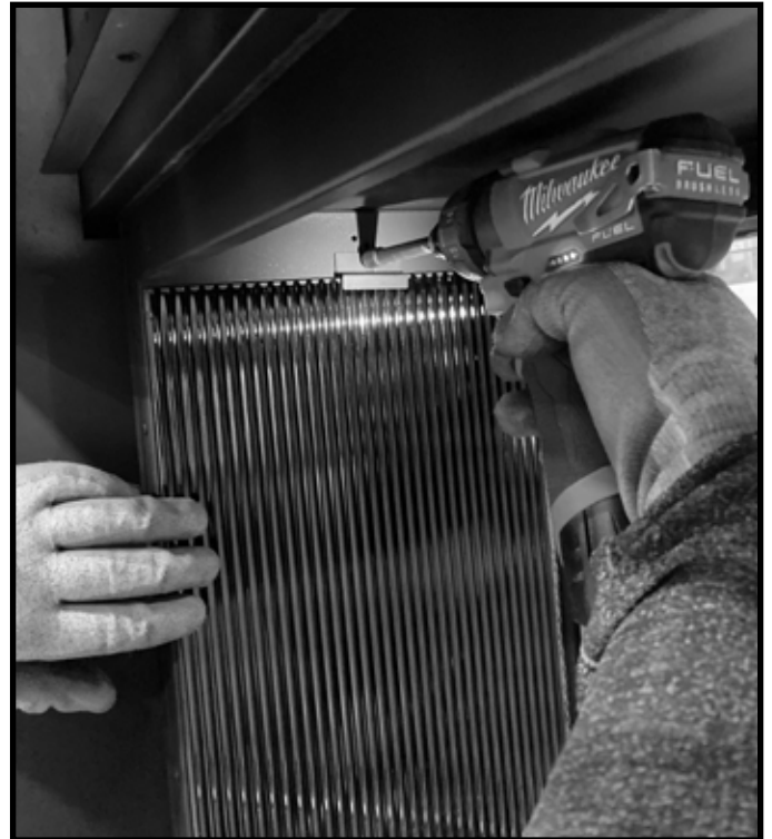
Figure 18 Install Side Panel Refractory Bracket
