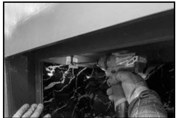
Figure 14 Install Refractory Bracket
