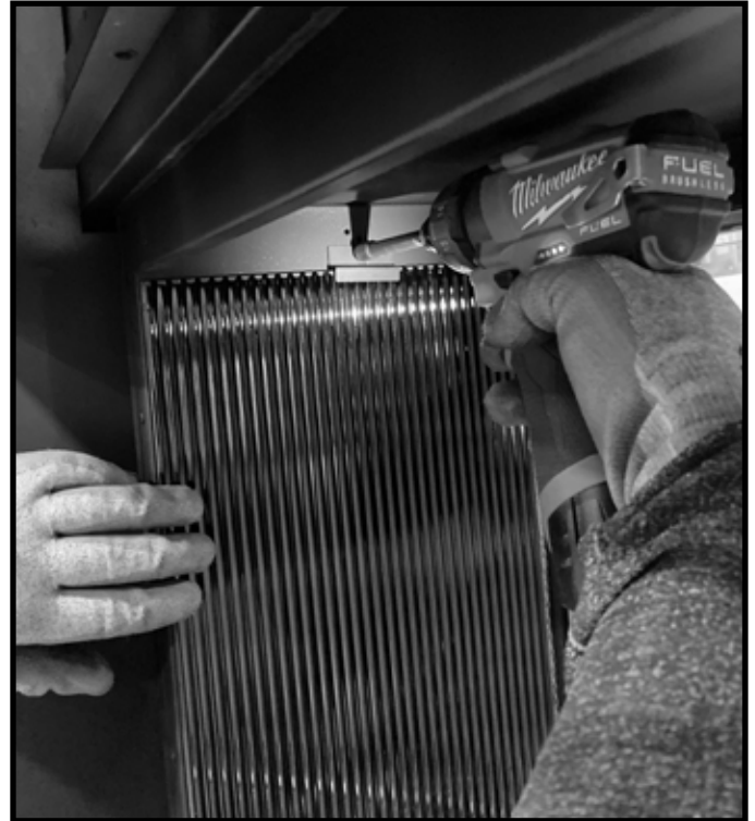
Figure 9 Installing Refractory Bracket with Self-Tapping Screw
