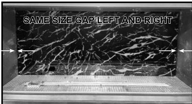
Figure 11 Gap is Equal on Both Sides
