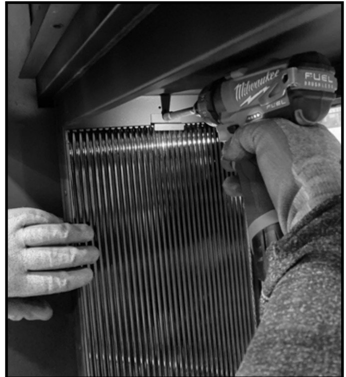
Figure 9 Installing Refractory Bracket with Self-Tapping Screw
