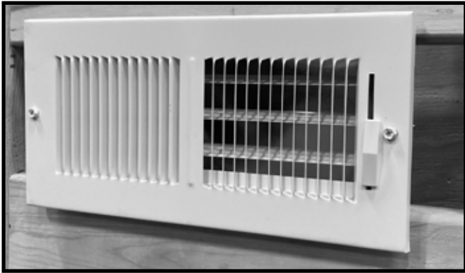
Figure 6 Register Cover Installed
