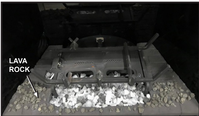
Figure 27 Lava Rock Installed (Example)
