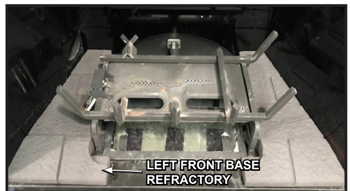
Figure 24 Left Front Base Refractory installed
