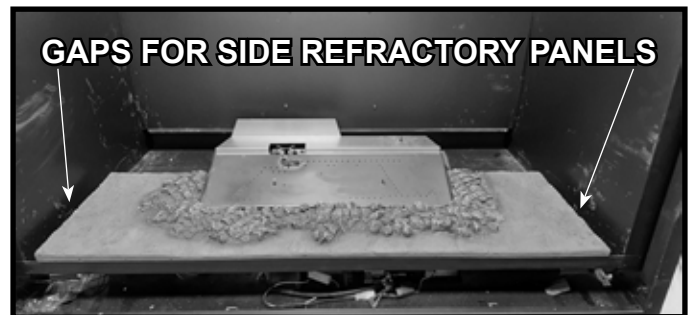
Figure 2 Base Refractory Installed
