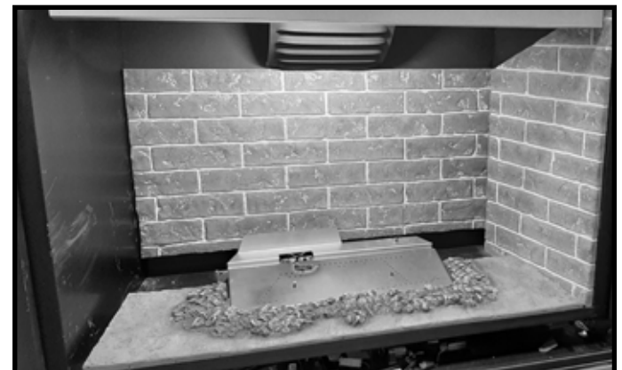
Figure 7 Side Refractory Panel Installed
