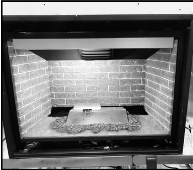
Figure 8 Refractory Kit Installed
