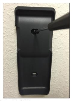
Figure 7 Install the Wall Mount
