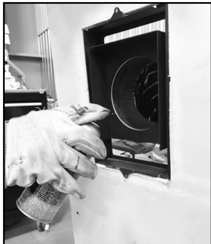
Figure 6.4 Paint Outer Wrapping of Flex Vent (Optional)
