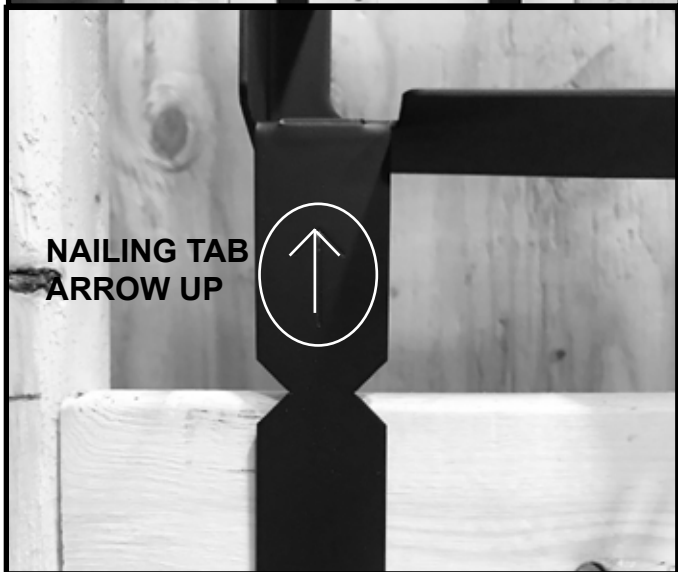
Figure 5.13 Side Discharge Assembly Nailing Tab Orientation
