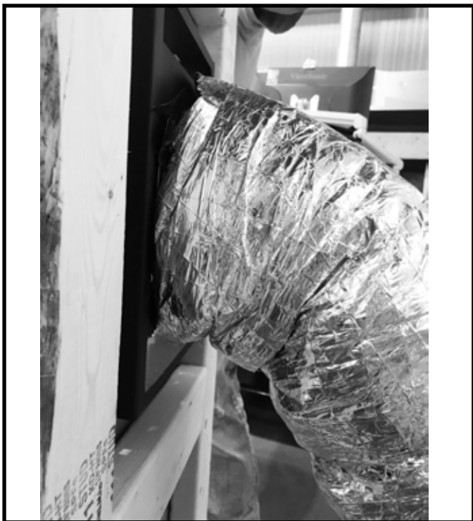
Figure 5.16 Install Flex Venting to Side Discharge Assembly
