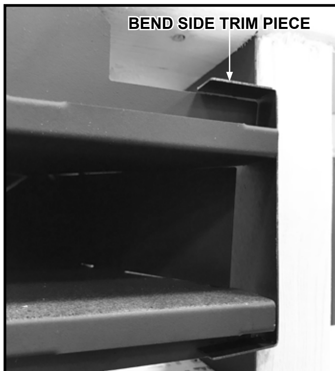
Figure 5.24 Bend Side Trim Piece
