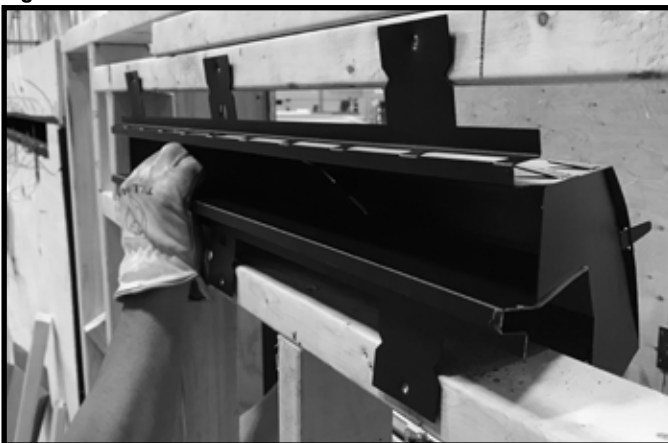
Figure 5.18 Position Plenum
