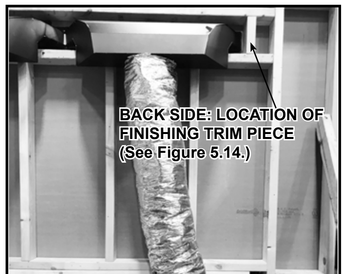
Figure 5.29 Flex Vent Installed with No Kinks
