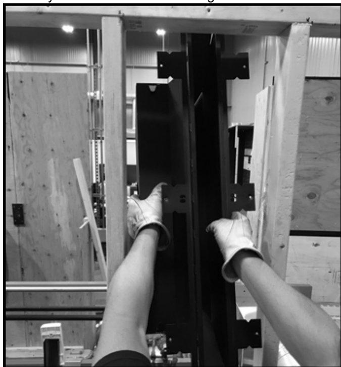
Figure 5.15 Turn Plenum Vertically to Clear Framing Studs
