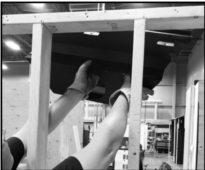
Figure 5.16 Rotate Plenum to Horizontal Orientation
