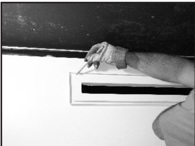
Figure 3 Mark Holes for Register Backer
