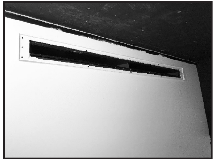
Figure 4 Register Backer Installed
