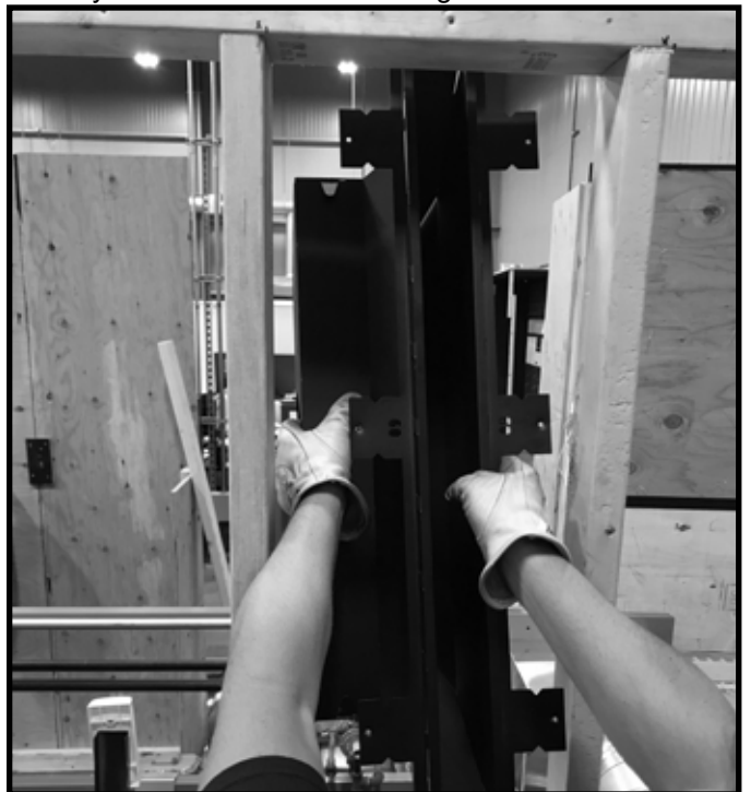
Figure 6.6 Turn Plenum Vertically to Clear Framing Studs
