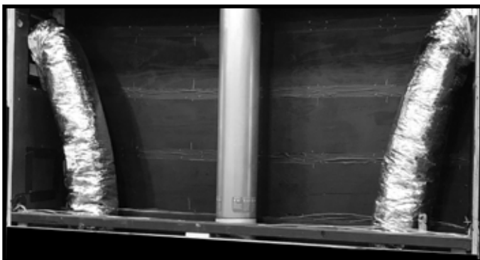
Figure 7.7 Flex Venting Installed
