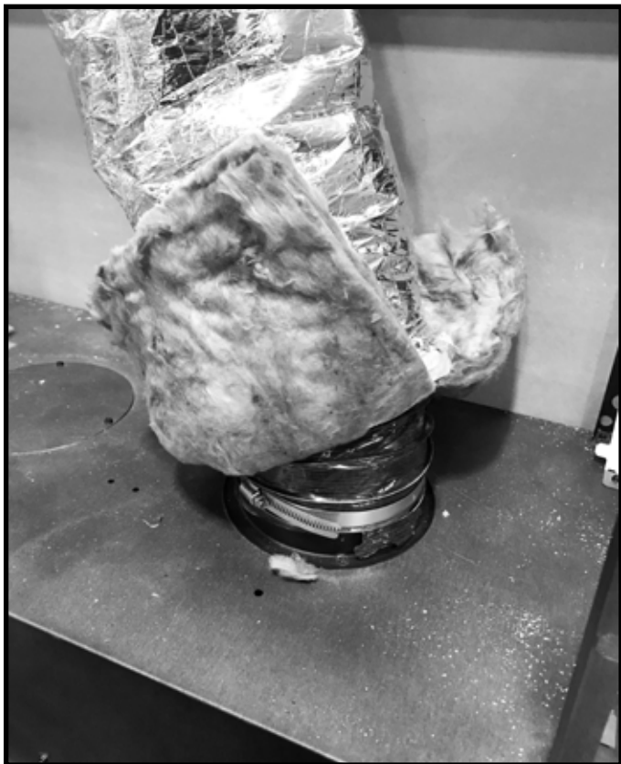
Figure 6.18 Install Flex Venting to Appliance
