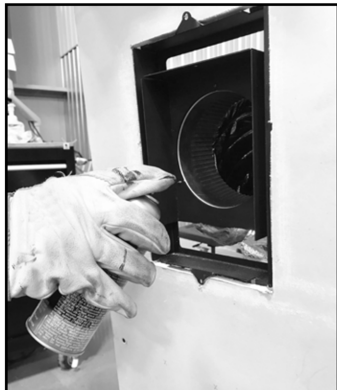
Figure 7.11 Paint Outer Wrapping of Flex Vent (Optional)
