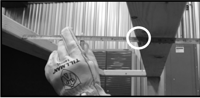
Figure 8.3 Measure Chase Depth
