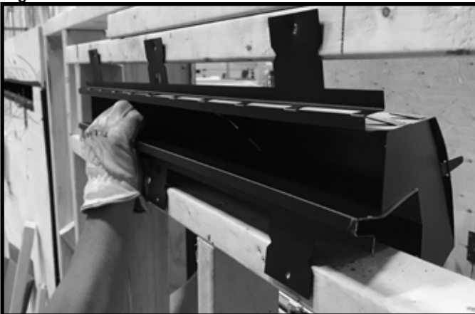
Figure 6.9 Position Plenum
