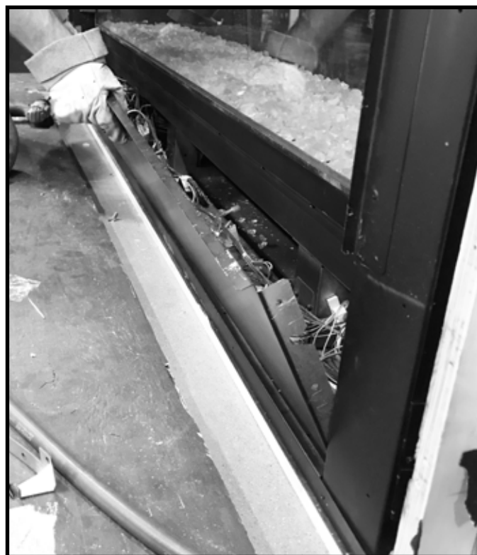
Figure 5.3 Remove Bottom Panel
