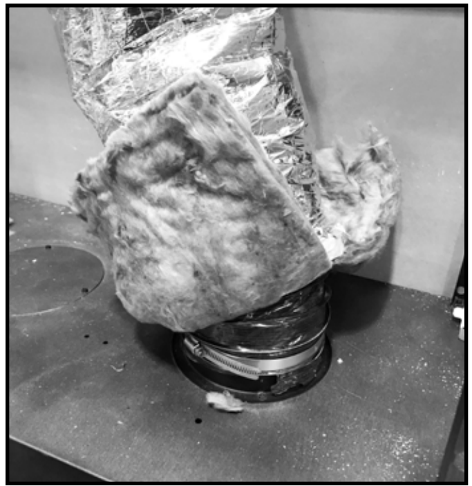
Figure 7.4 Install Flex Venting to Appliance
