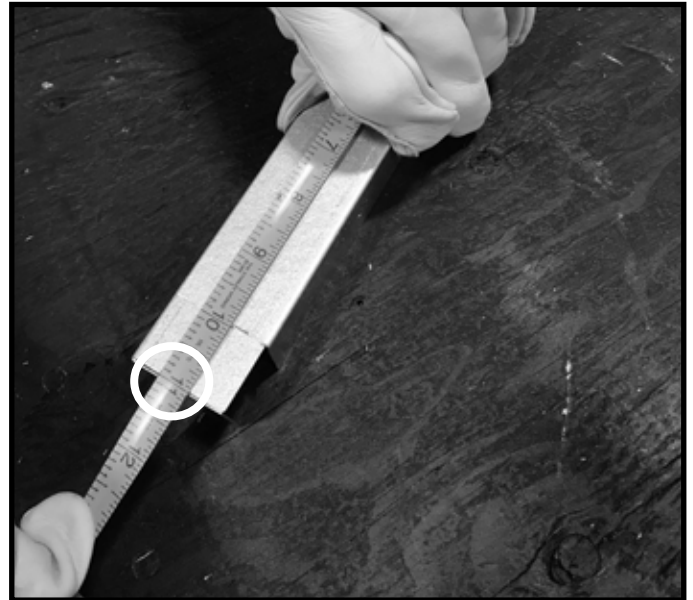
Figure 8.5 Measure Length of Mounting Brackets
