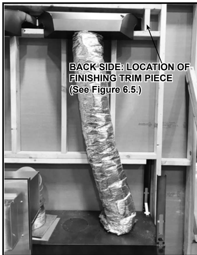
Figure 6.20 Flex Vent Installed with No Kinks
