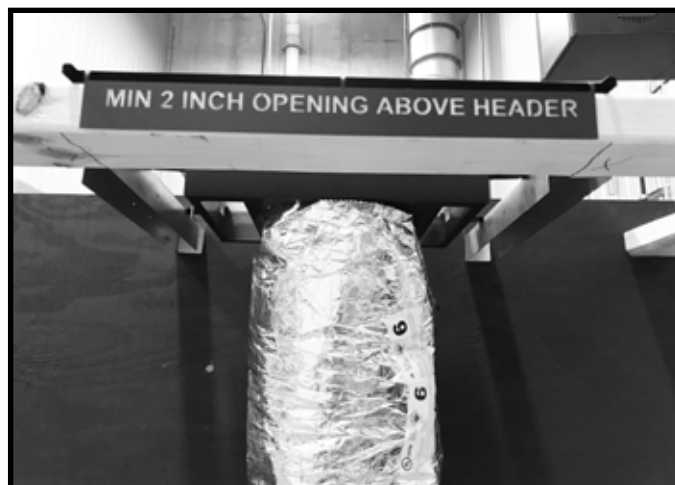
Figure 8.23 Install Flex Venting to Appliance
