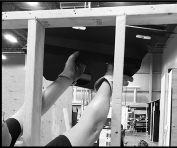
Figure 6.7 Rotate Plenum to Horizontal Orientation
