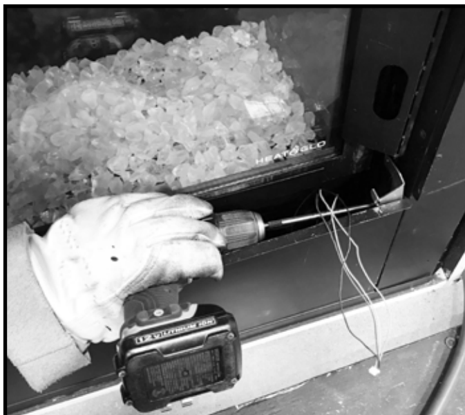
Figure 5.2 Remove Existing Glass Mounting Brackets (If Installed)
