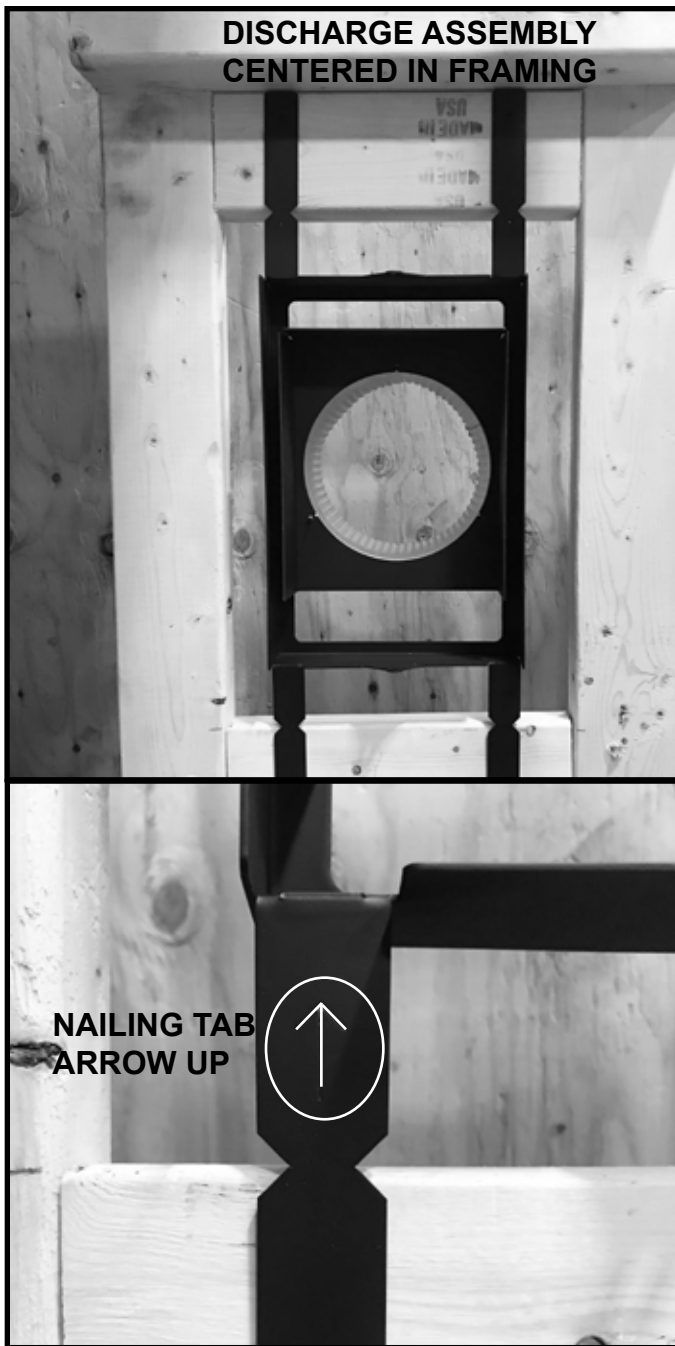
Figure 7.3 Side Discharge Assembly Nailing Tab Orientation
