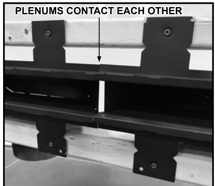
Figure 6.12 Plenums Contact Each Other
