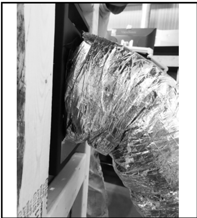
Figure 7.6 Install Flex Venting to Side Discharge Assembly
