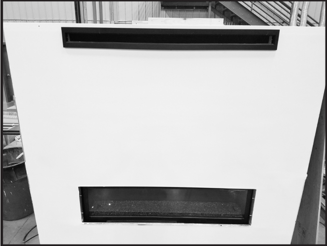
Figure 6 Vent Cover Installed
