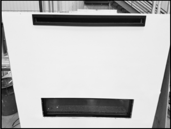
Figure 6 Vent Cover Installed
