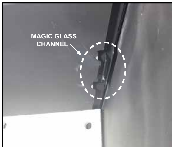
Figure 5 Location of top Magic Glass channels
