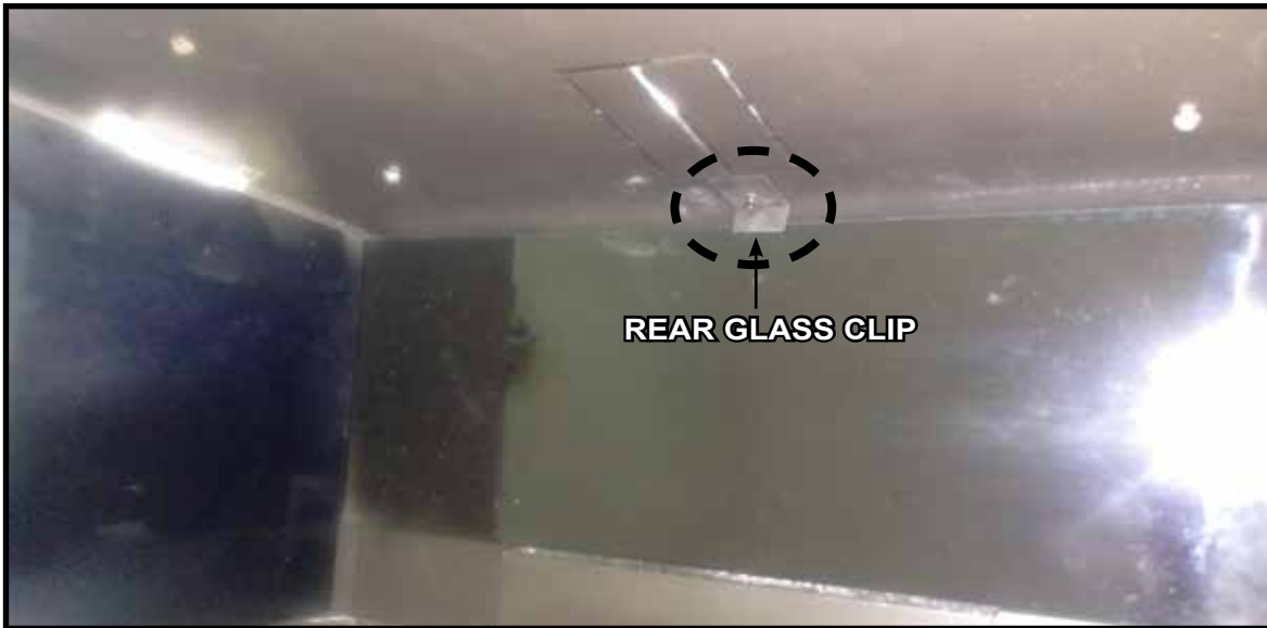
Figure 6. Install Rear Glass Panel
