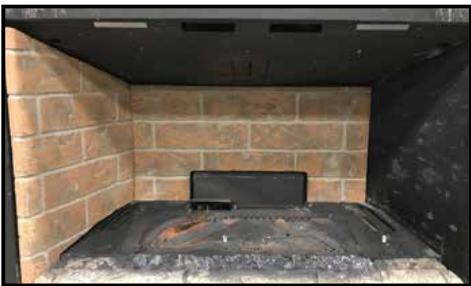
Figure 7 Left Refractory Installed
