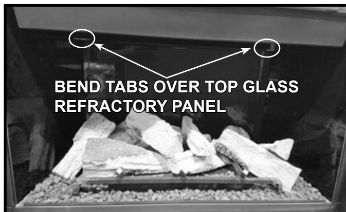
Figure 11. Glass Refractory Installed
