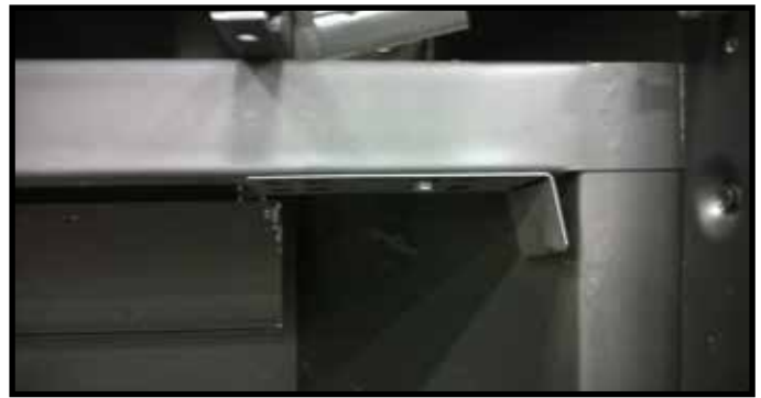
Figure 5. Glass Refractory Brackets Installed
