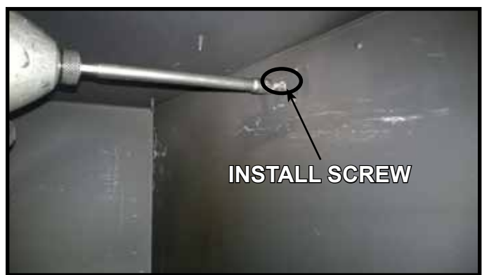
Figure 1. Remove Fiber Refractory Brackets. Install Screw.
